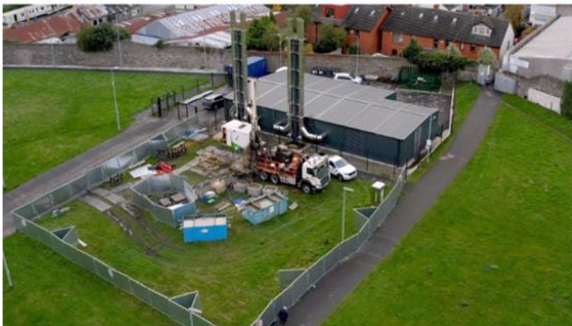
Figure 23 – Borehole at TUD
